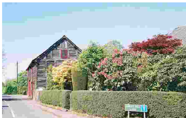
Coppice Farm Barn on Ashley Mill Lane.
